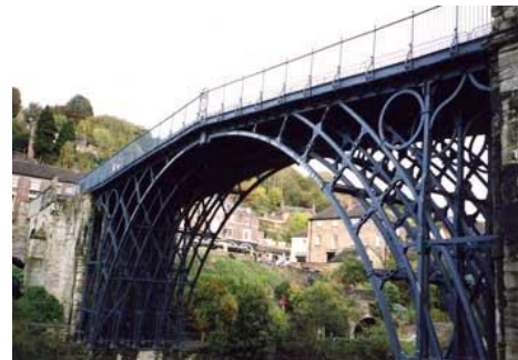
Fig. 12 The Iron Bridge made from non-chilled flake graphite cast iron, in 1799 (World's Cultural Heritage in Coalbrookdale, UK)
