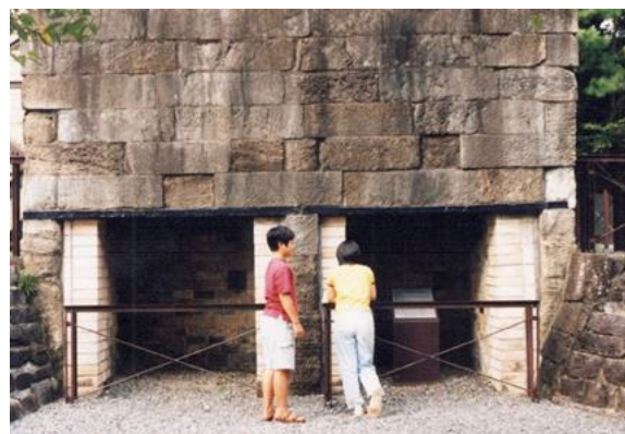
Fig. 16 Entrance of air into firebox
