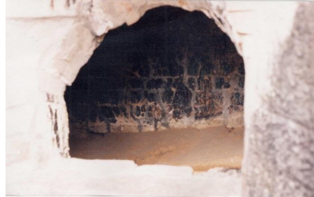
Fig. 18 Holes to put metal materials onto fire grate and to put fuel into firebox
